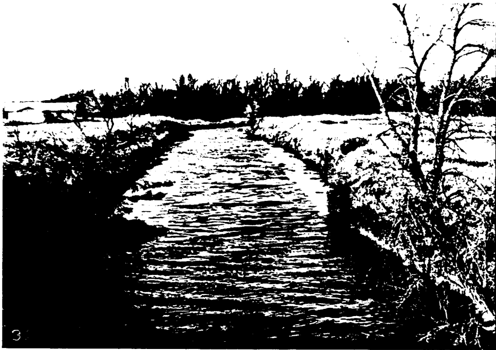
Julesburg Reservoir Inlet Canal
