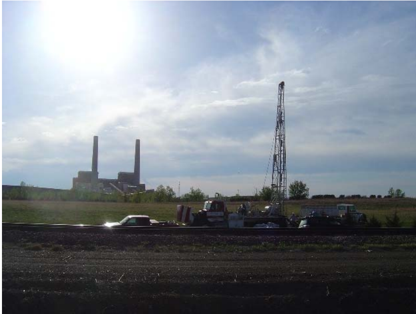
IMAGE 4. Drill site of geochemical monitoring well nest 6, east of GGS. Drill cuttings from this borehole provided lithologic data from the middle of the well field. Photo taken in May 2006.
