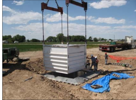
Figure 5. The inner tank plus soil being lowered inside the containment tank
