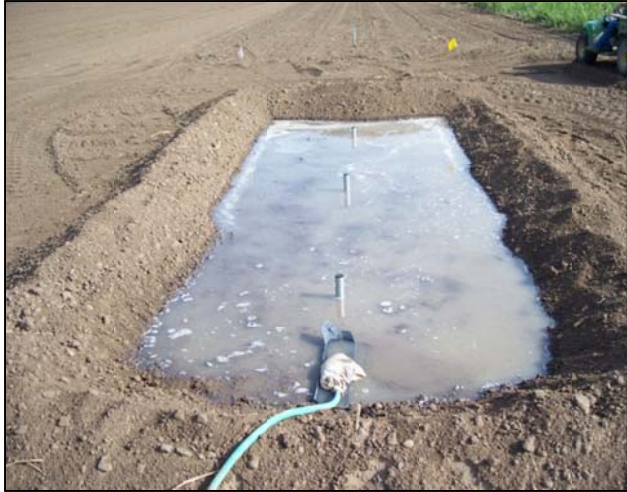
Figure 16. Water being added to the 'wet' set of neutron probe access tubes. The 'dry' set is in the background. Photo by Lane Simmons
