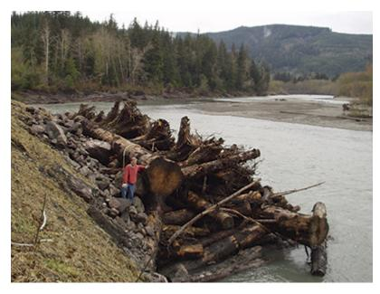
Figure 4. An example of a large engineered logjam built by the Washington State Department of Transportation on the bank of the Hoh River along U.S. Highway 101.
