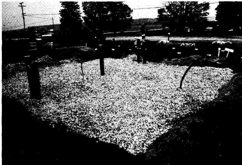
Fig. 7. Place the stones in the bed to a depth of 9 in. and level the stones.
