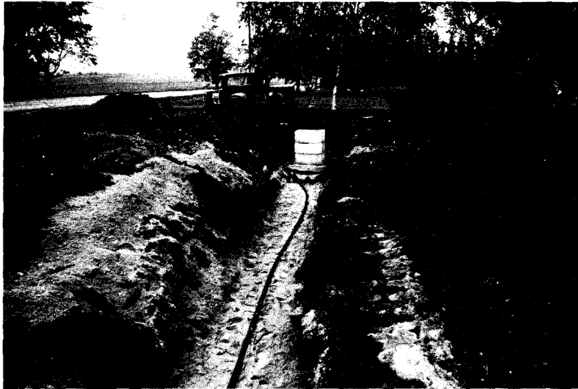
Fig. 3. Trench and lay the pipe from the pumping chamber to the fill system. Normally a 1\frac{1}{2} to 2 in. PVC, schedule 40 or 80, pipe is recommended.
