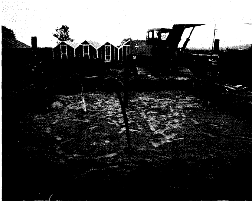
Fig. 6. Placement of bed in the fill system. This can be done with crawler tractor with blade. Bottom must be level, thus requiring some hand leveling.
