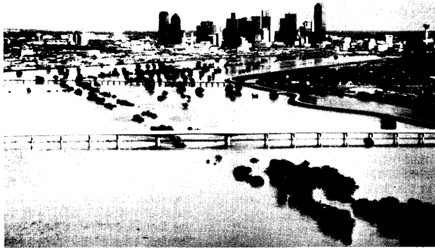
Photo 2. The Trinity River is out of its banks along the Dallas Floodway at a near record level on May 3, 1990. (Courtesy Fort Worth District, U.S. Army Corps of Engineers, Ron Ruffennach).
