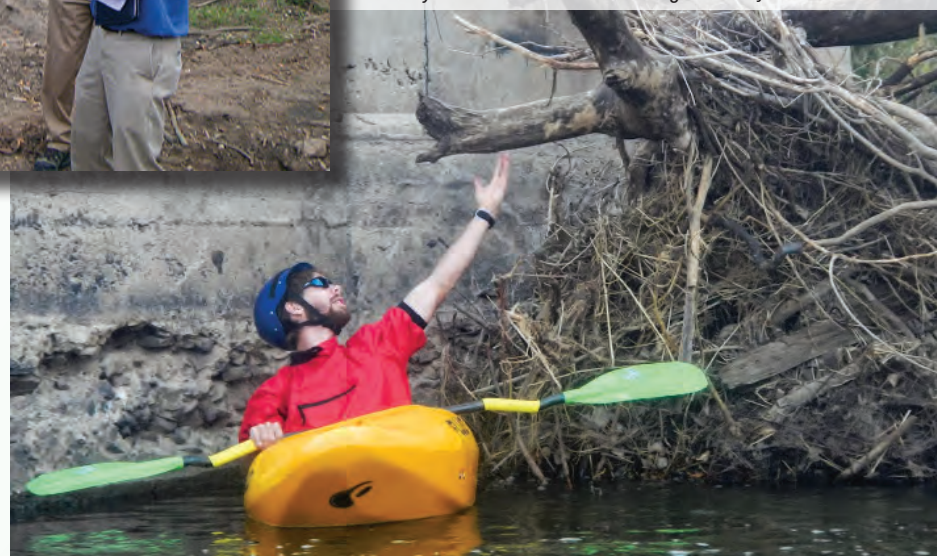
Wood piled against a train bridge pier on the Poudre River near Greeley after the Fall 2013 flooding. Photo by Natalie Anderson
