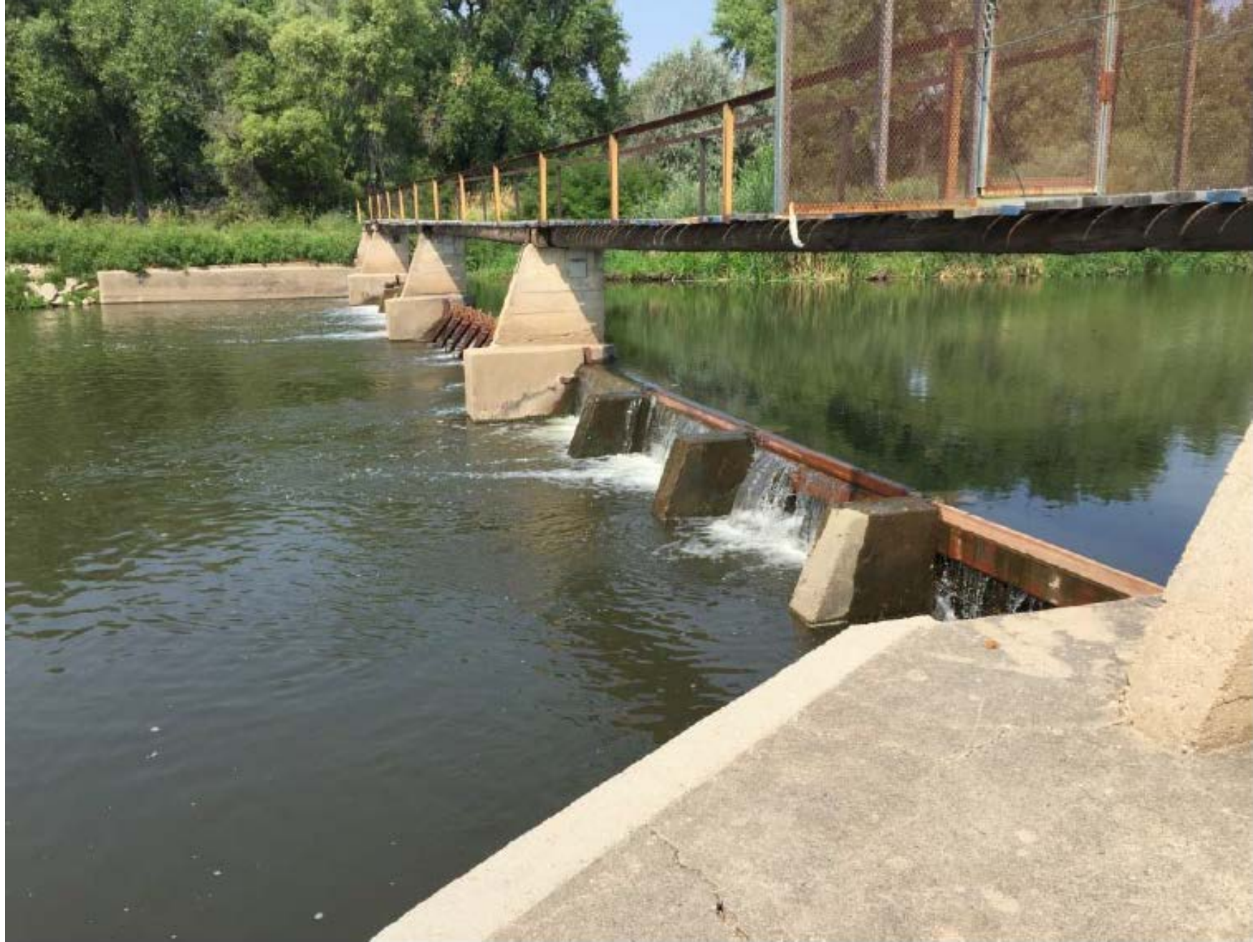
Figure 10 – Whitney Diversion Structure
