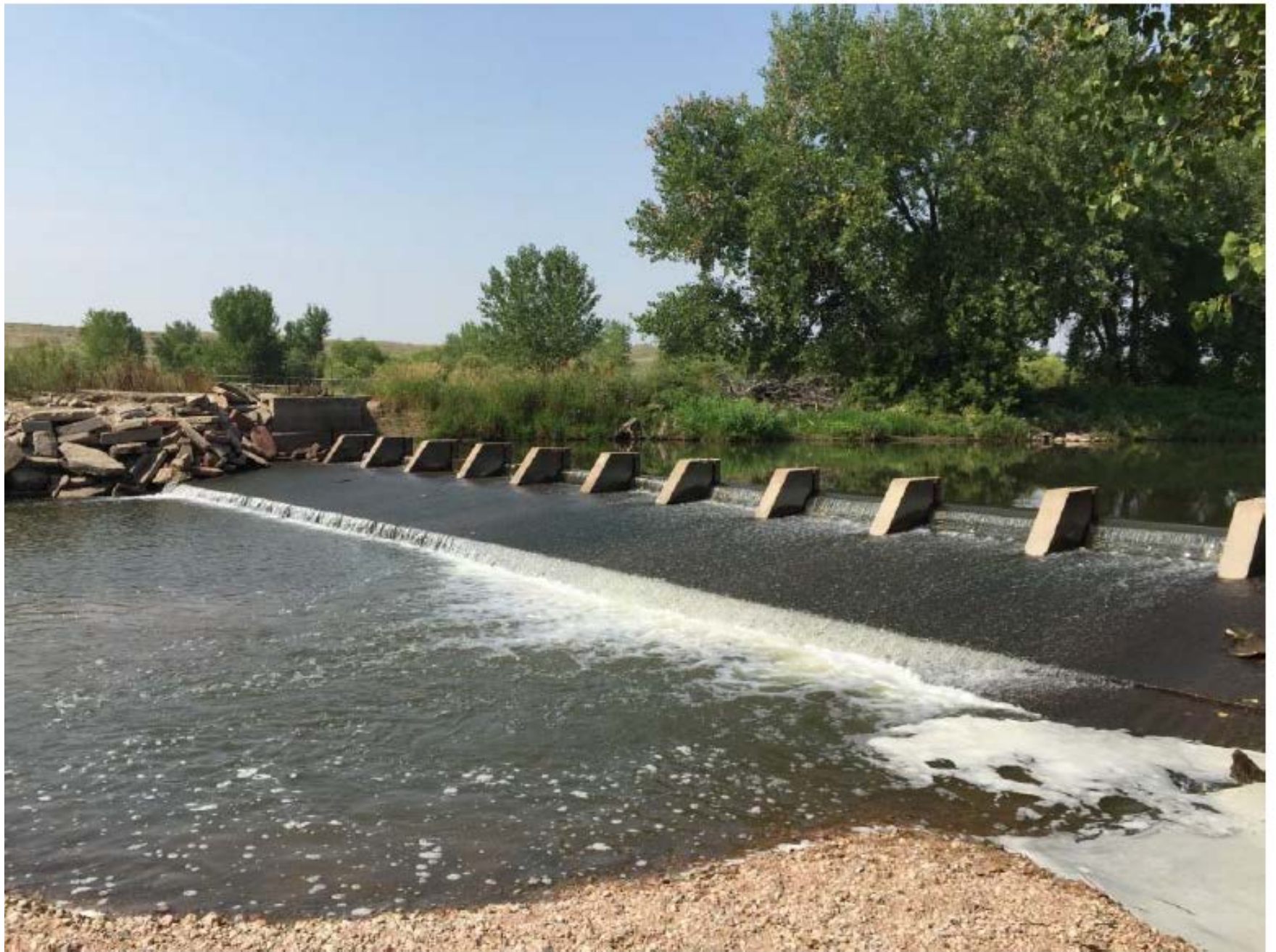
Figure 11 – BH Eaton Diversion Structure
