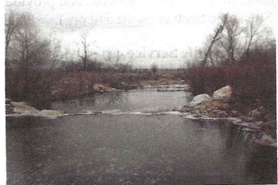
BOULDER CROSS-VANE DIVERSION
