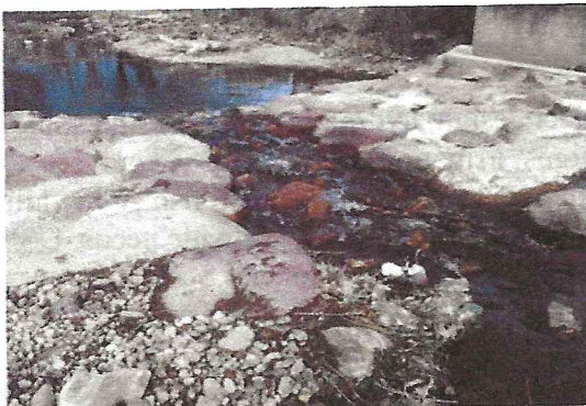
TRADITIONAL DIVERSION WITH ROCK RAMP
