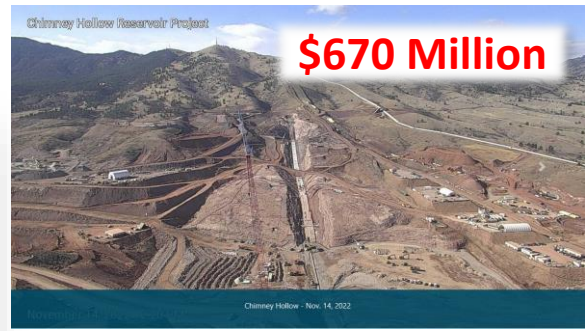
Chimney Hollow Construction 350 ft tall dam, 90,000 acre-ft
