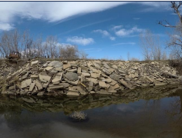
Concrete Rubble & Debris Lined Banks
