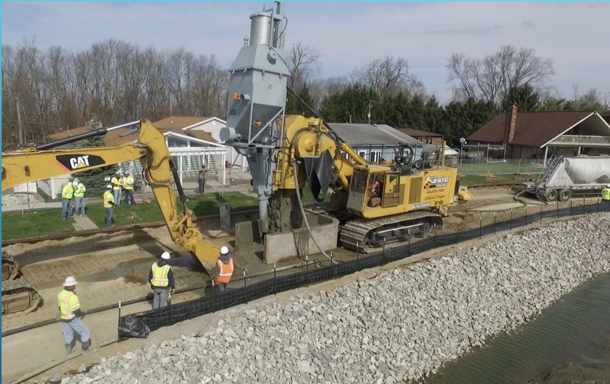
PHOTO FROM DEWIND ONE-PASS TRENCHING
