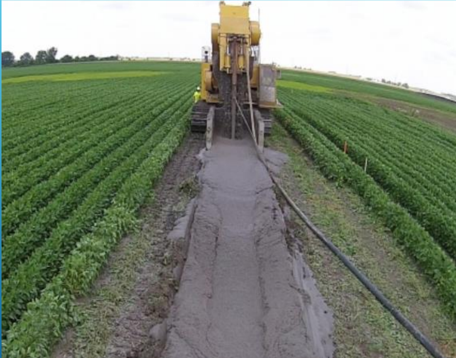
PHOTO FROM DEWIND ONE-PASS TRENCHING
