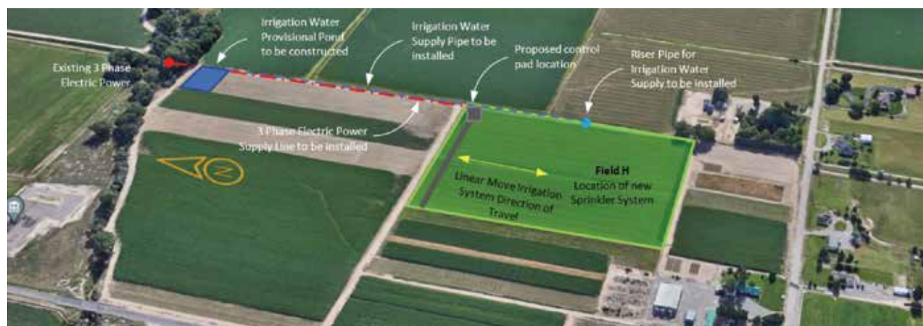
Figure 1. Aerial view of the Western Colorado Research Center at Grand Valley field where Overhead Linear Move System is being installed.
