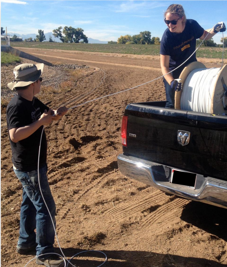
Installing fiber optic cable
