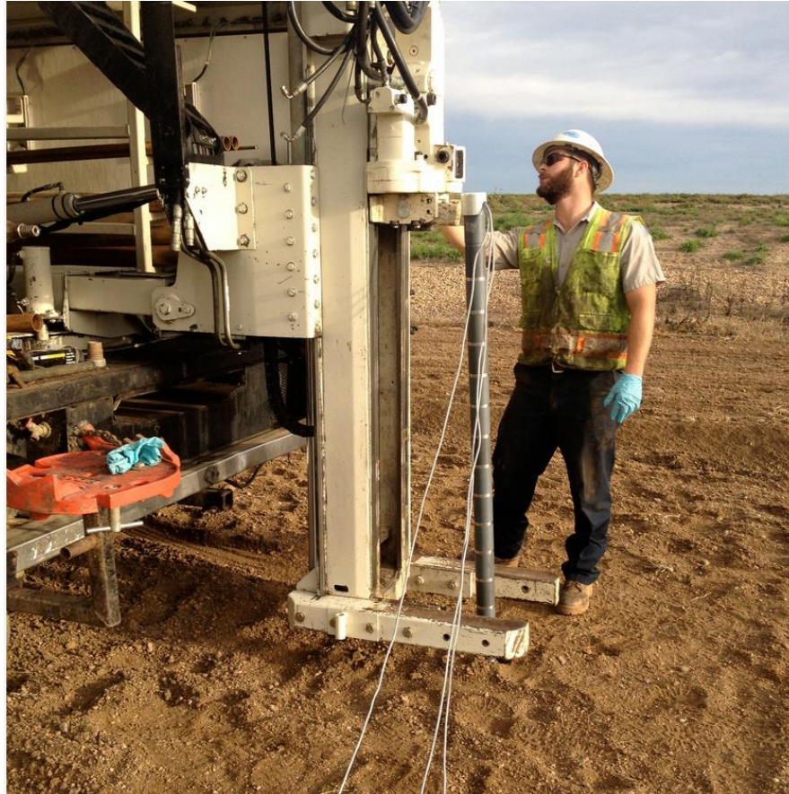
Installing vertical resistivity probe in MAR basin
