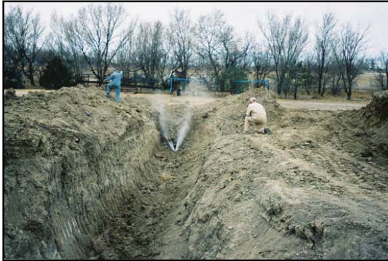
Jet Cleaning of Tile Lines: Photo shows a jet nozzle working through a tile line that has been plugged for many years. The current study estimates that there are approximately 140 miles of old tile lines in the lower Arkansas Valley that need maintenance work of this nature.
