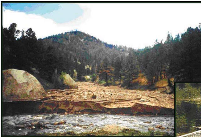
STRONTIA SPRINGS RESERVOIR AFTER THE BUFFALO CREEK FIRE: These photos show the damage that occurred after heavy rains washed debris into Strontia Springs, a major water source for the Metro Denver area. The area was burned during the Buffalo Creek Fire. Denver Water has spent millions of dollars dredging the reservoir and removing debris.
