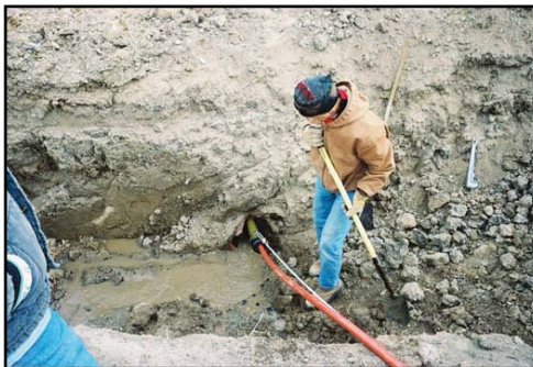
Jet Cleaning of Tile Lines: Modern sewer maintenance technology is very well suited to maintaining buried tile lines throughout the lower valley.
