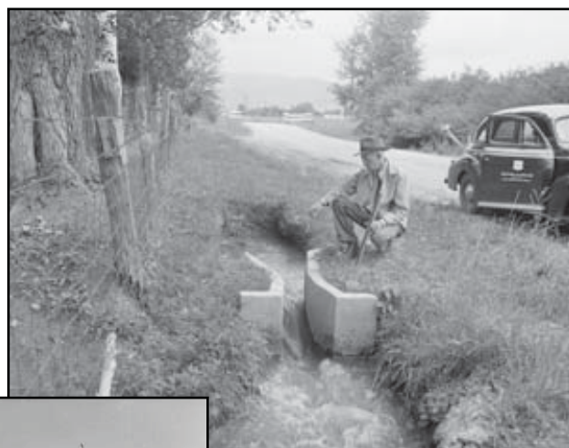
TOP: Parshall takes measurements using his invention, the Parshall Flume, 1932, from the Ralph L. Parshall Collection, Water Resources Archive, CSU.
