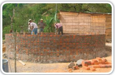
A 25,000-gallon tank is constructed in the community of Union Otuta, Santa Rita. On top of the completed tank is the drip chlorination device used for disinfection.
