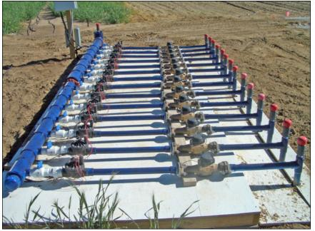
*This valve and flow meter manifold is used to control and measure irrigation applications. (Courtesy of Thomas Trout)*
