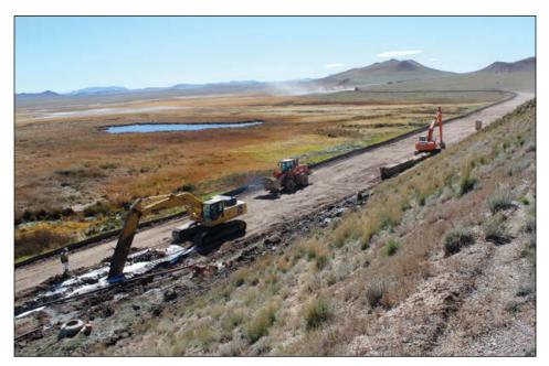
Crews build a sand trench on the downstream side of Antero Dam to filter the normal seepage of the dam and to stabilize the foundation. Photo by Ann Baker
