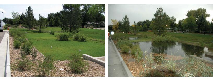
Figures 3 and 4. Bioretention cell installed in Fort Collins, CO during dry and wet weather. Bioretention cell treats stormwater runoff from an adjacent parking lot. Photos by Chris Thornton
