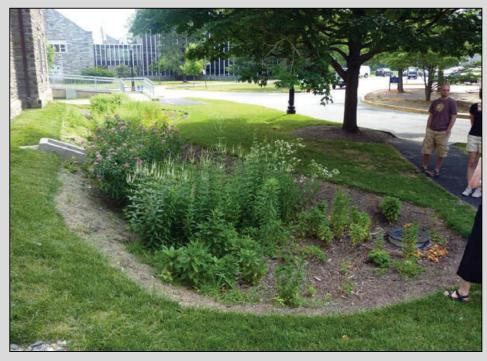
Figure 6. Raingarden collects roof and driveway runoff and infiltrates it into ground. Notice the storm inlet at the lower right to drain off runoff from larger storms.
