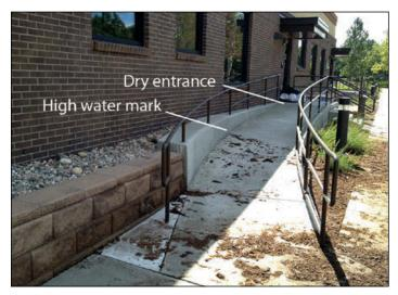
Figure 2. Debris line is evident on west side of Orthopedic Center of the Rockies showing the water level against the building. Approximately 6 inches of freeboard remained before water would enter the building, making this a good example of the benefits of elevating structures to protect from flood damage. Courtesy of City of Fort Collins Utilities
