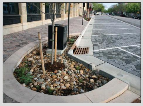
Figure 7. Modular pavement and infiltration basin.
