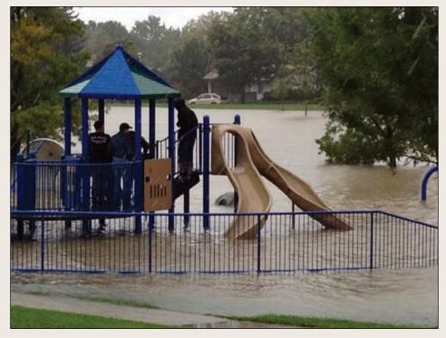
Utah Park in Aurora, Colorado is a detention basin that worked as designed to minimize damage from floodwater to neighboring property during the September, 2013 flooding. Photo by Jeremy Deischer
