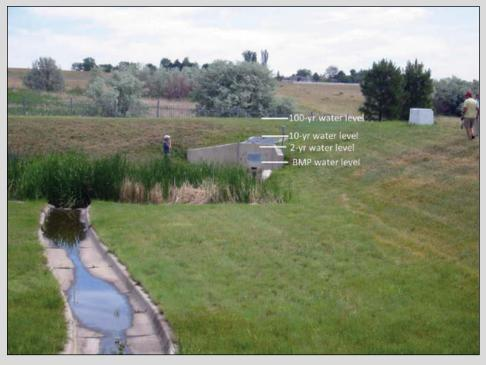
Figure 5. Typical stormwater detention facility providing peak flow attenuation and pollution removal.
