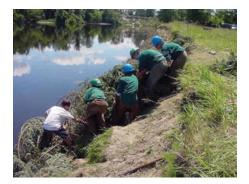
Workers along the Connecticut River as it passes through Fairlee, Vermont, United States. During the summer of 2002 a restoration project aimed at restoring a severely eroded riverbank utilized overgrown Christmas trees to create a revetment at the work site. The trees were eventually planted with various aquatic plant life to help further trap sediment and prevent erosion. Courtesy of US Environmental Protection Agency
