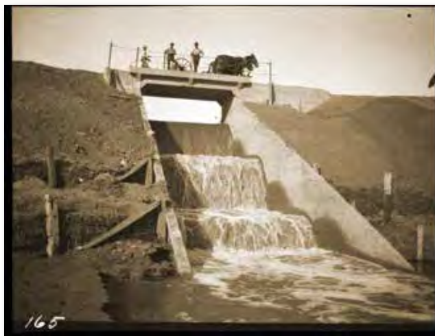
Drop structure in Satanta Canal, c. 1907-08.
